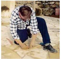
Measure the barrier according to your pool. Line up the posts and mark the holes.
