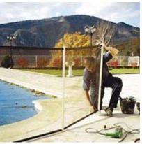
Insert the first post in the plastic sleeve. Tension the lower stripe and mark the next post hole. Drill the second hole and insert the next post in place. Follow same steps for all the other posts.
