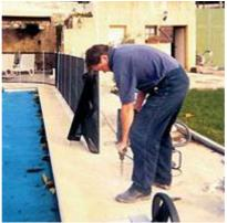
Drill the hole with 16 mm drill bit. Vacuum the dust from the hole and insert the post into the lock in deck feature.
